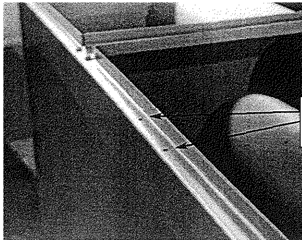
HOLES FOR FAN LIMIT CONTROL
