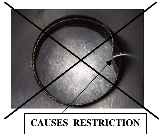
FAULTY INSTALLATION
